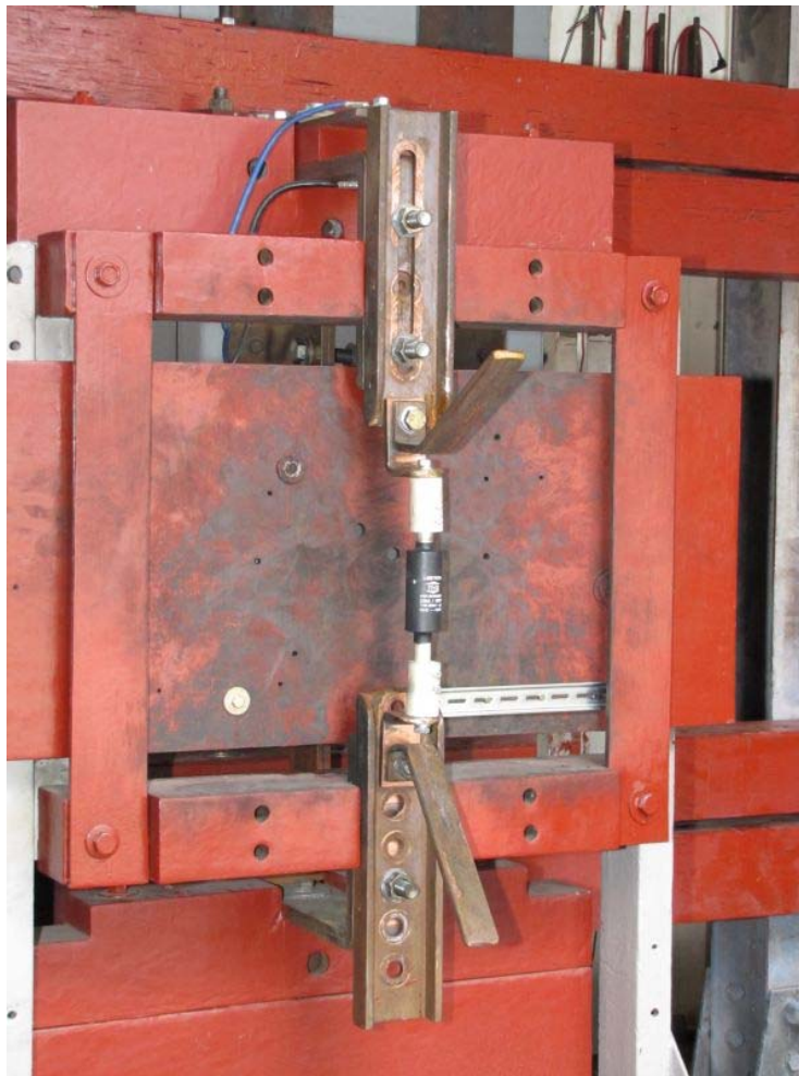
Photo 3: Test arrangement with fuse THS 250
